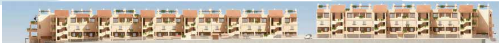
VIEW OF THE BACK FAÇADE
